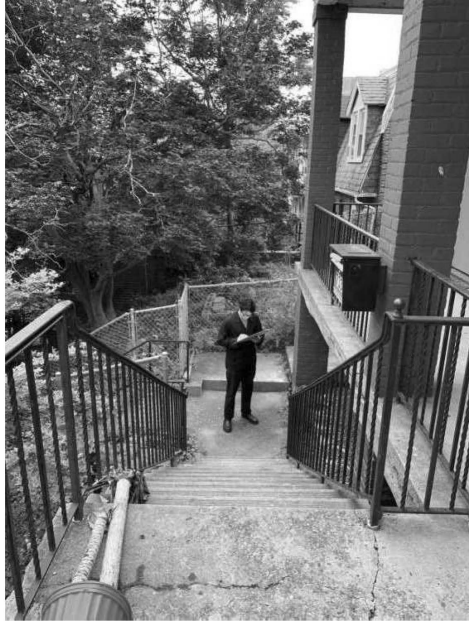
STEPS DOWN TO FRONT GRADE LEVEL
